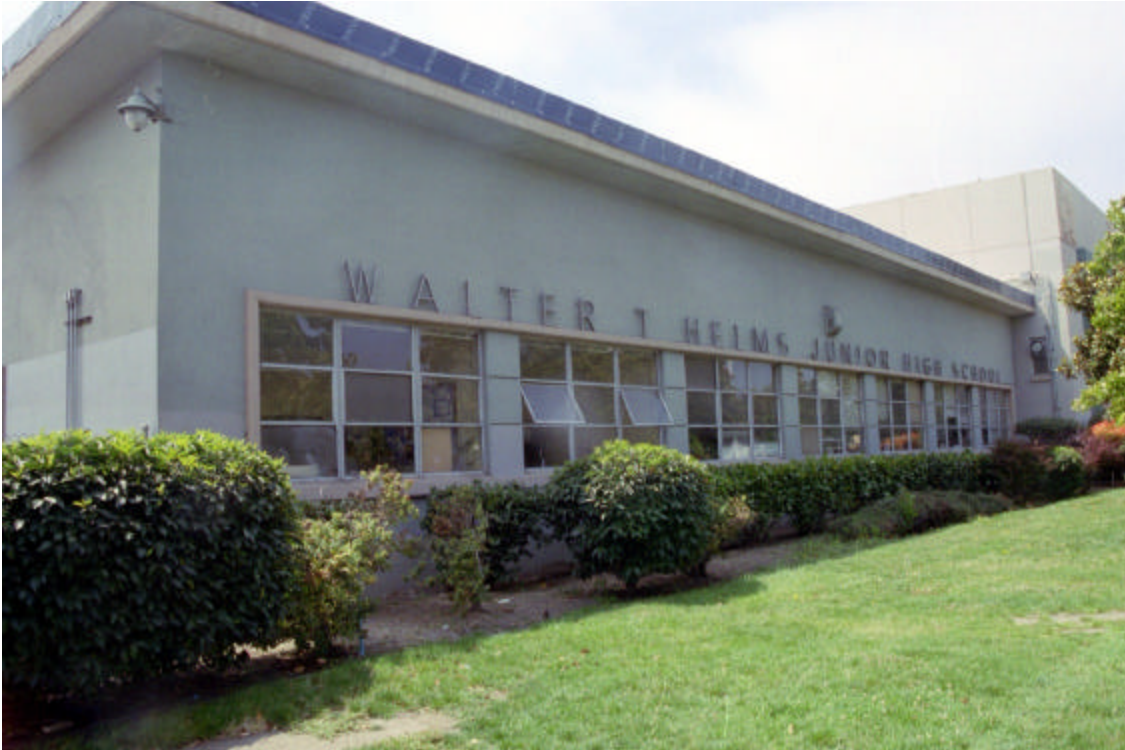
Figure 2: Main Building, administration wing, exterior north wall
