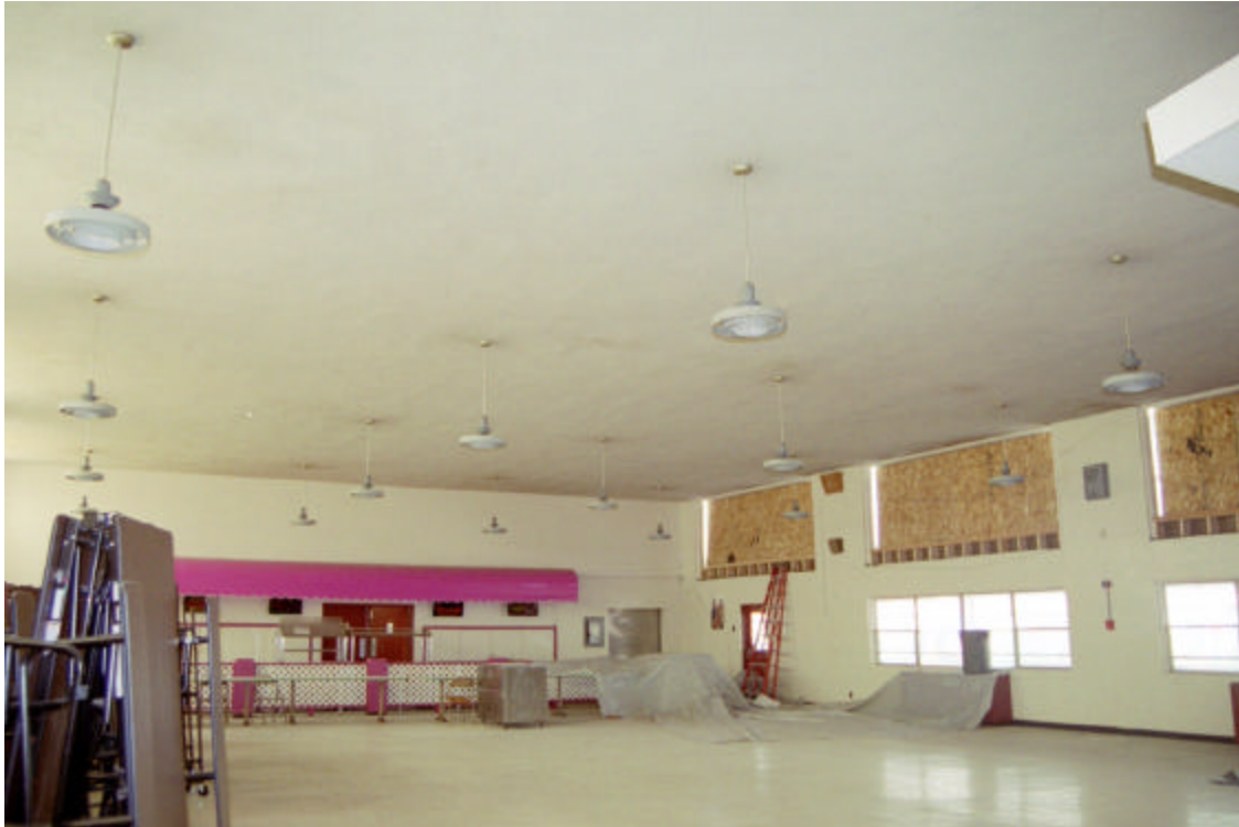
Figure 12: Main Building, wing 5, interior at cafeteria
