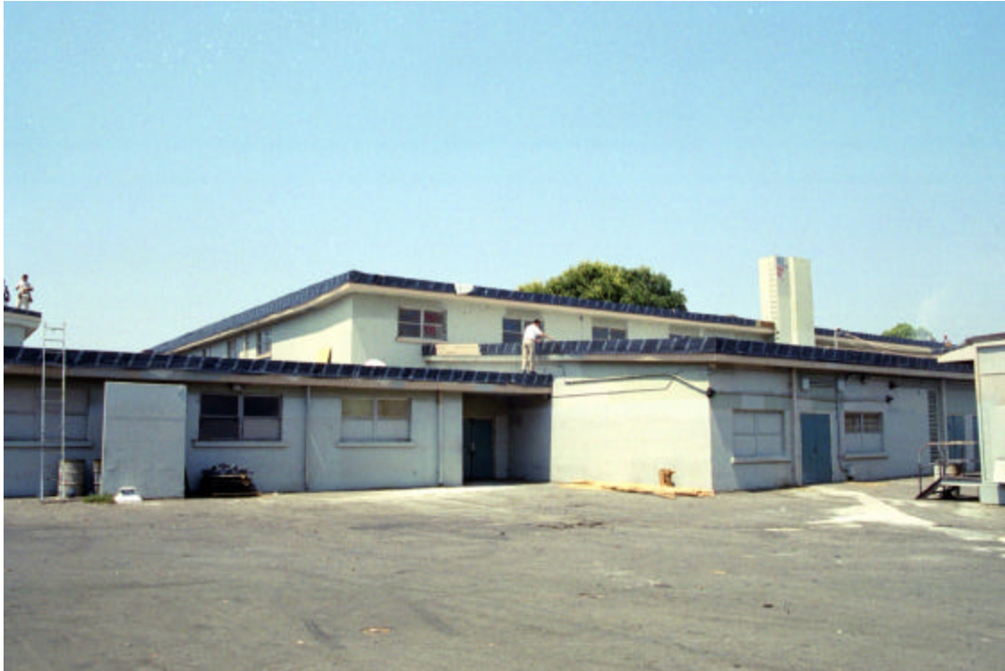
Figure 8: Main Building, exterior east wall at boiler room
