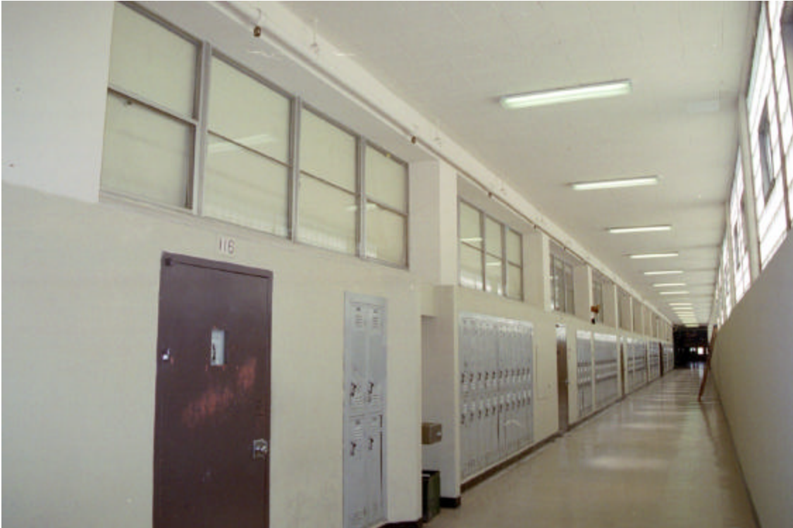
Figure 10: Main Building, classroom wings, interior at corridor
