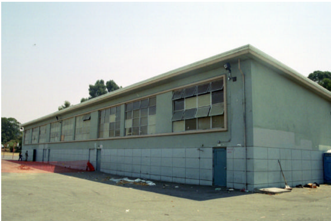
Figure 19: Shop Building, exterior north wall
