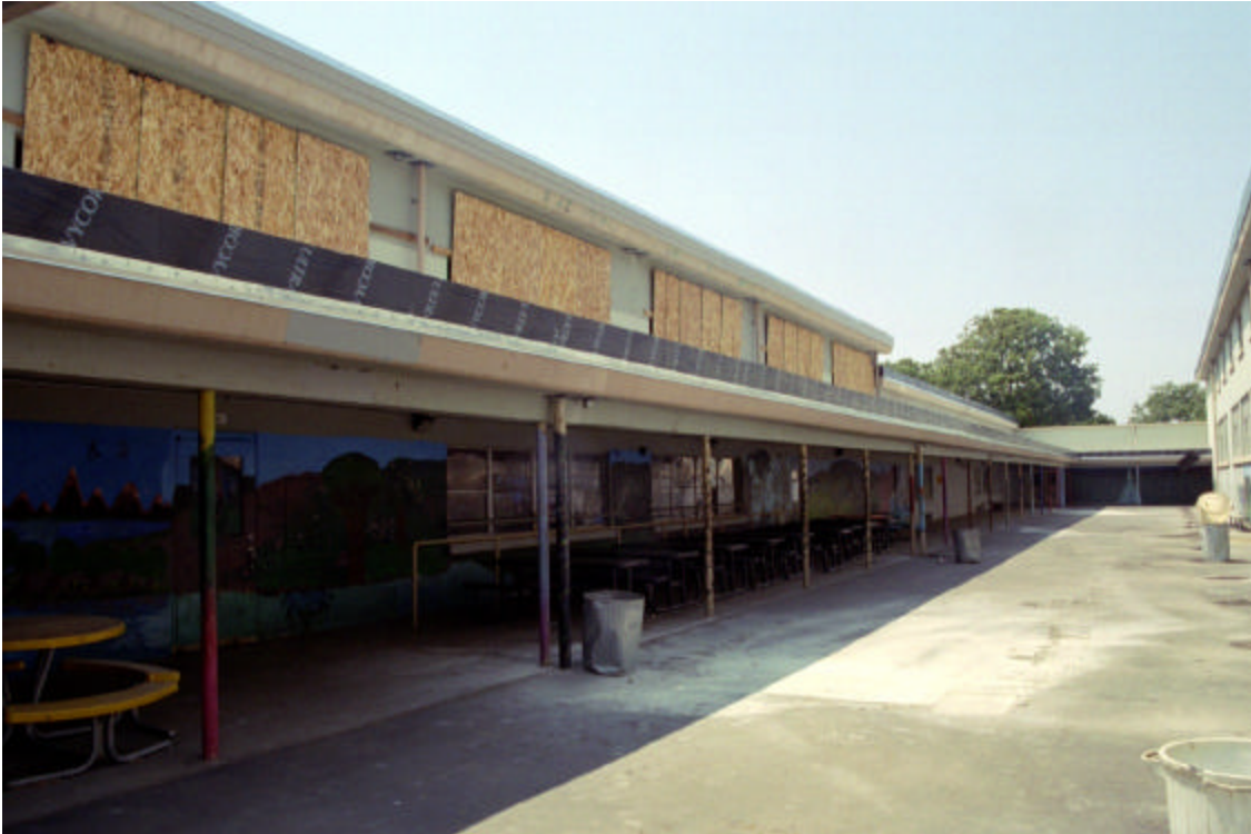
Figure 7: Main Building, wing 5, exterior north wall
