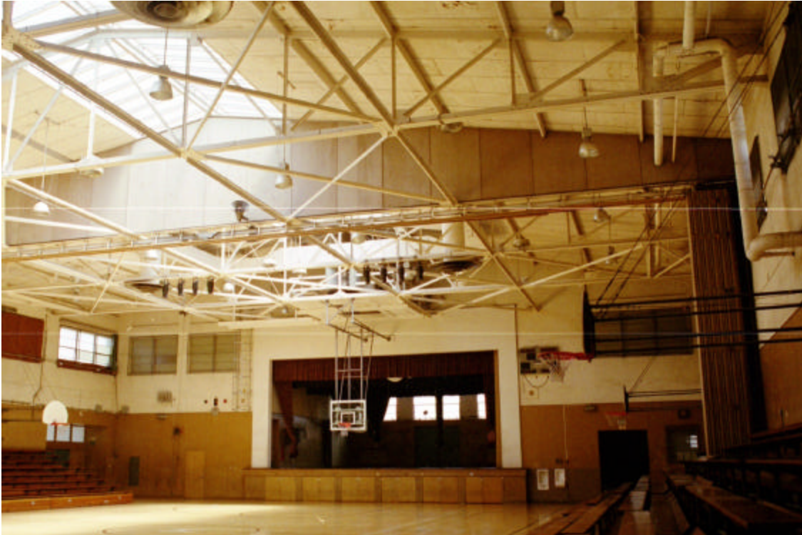
Figure 17: Gymnasium Building, interior at main gym area
