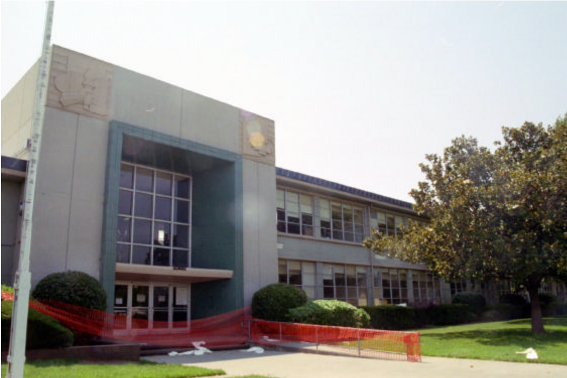
Figure 3: Main Building, wing 1, exterior north wall
