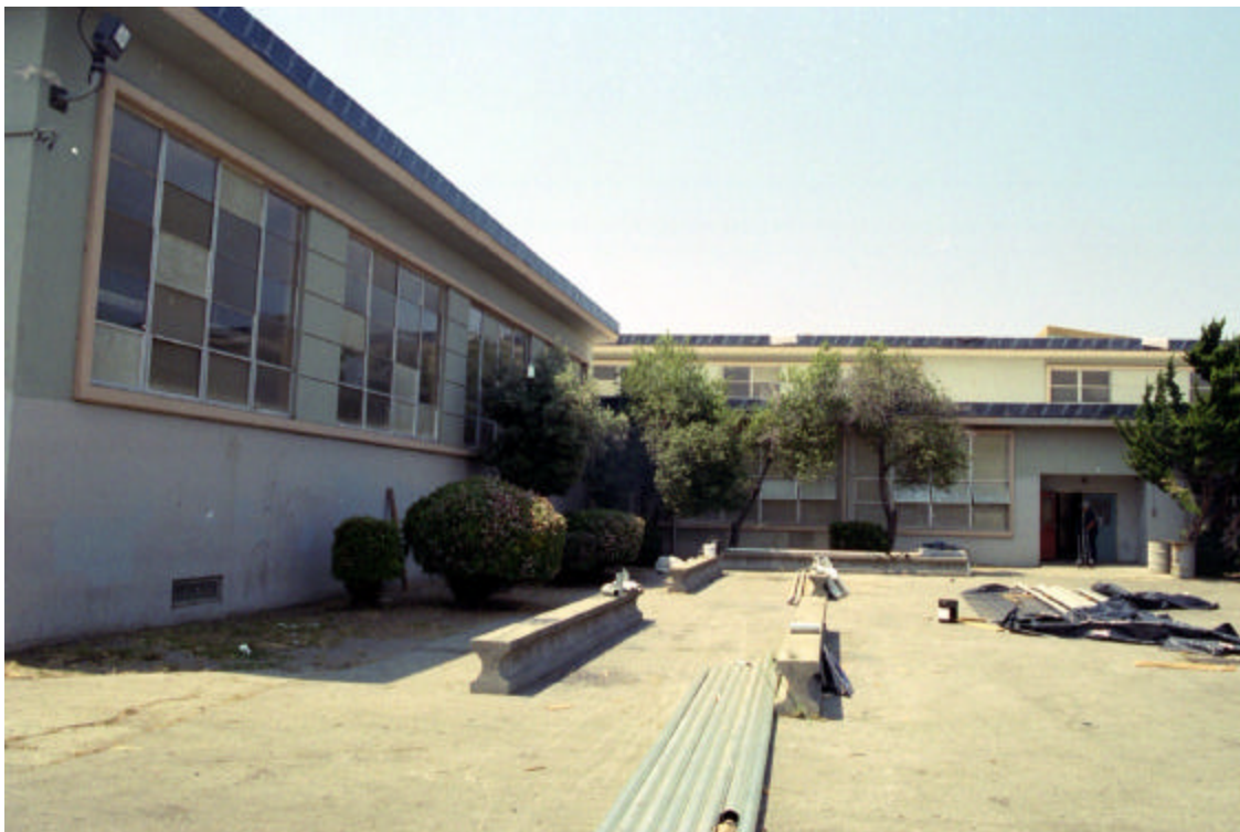
Figure 9: Main Building, library wing, exterior north wall
