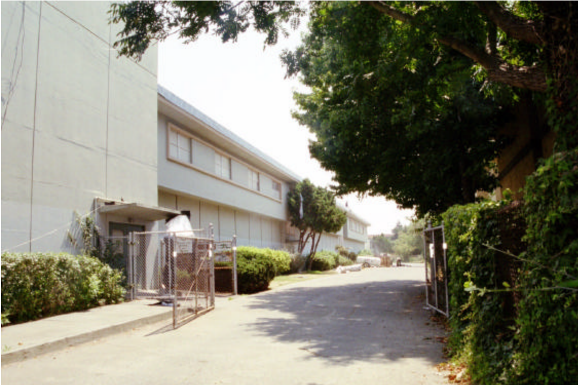
Figure 4: Main Building, exterior west wall
