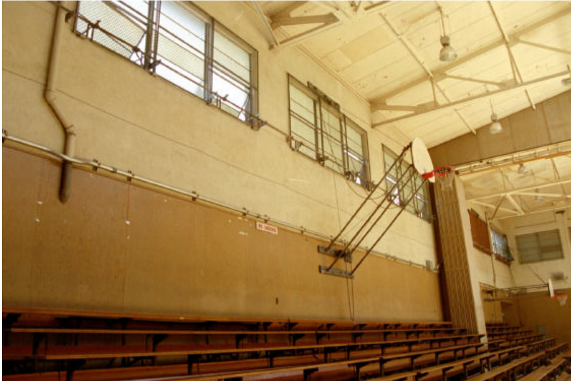
Figure 18: Gymnasium Building, interior at north wall of main gym area
