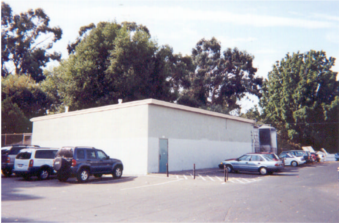
Figure 22: Music Building, exterior northeast corner
