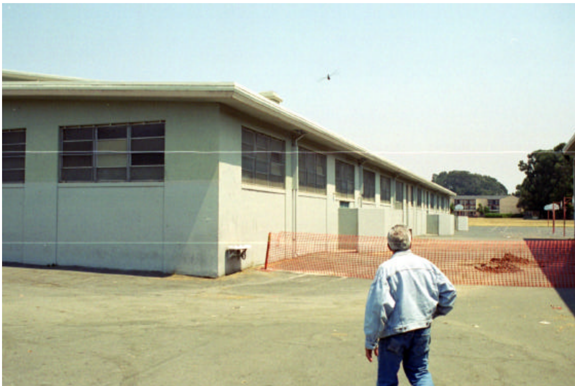
Figure 15: Gymnasium Building, exterior southwest corner
