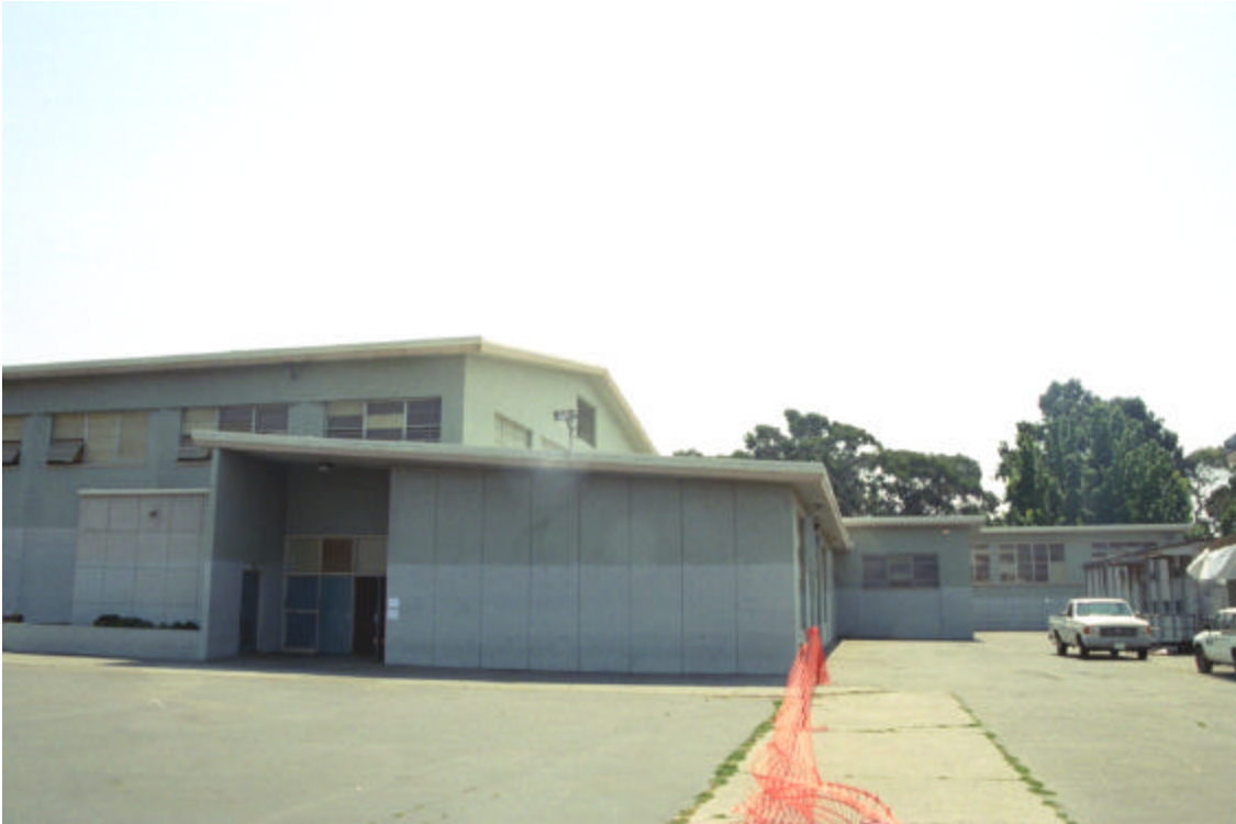
Figure 16: Gymnasium Building, exterior northwest corner
