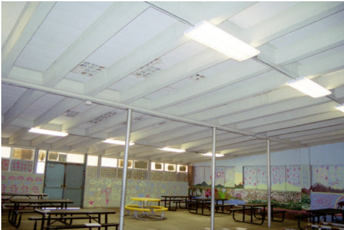
Figure 13: Main Building, wing 5, interior at additional dining area
