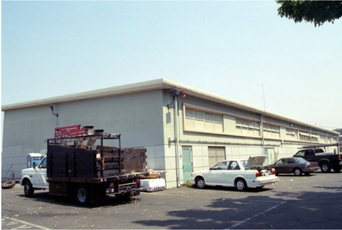
Figure 20: Shop Building, exterior southwest corner
