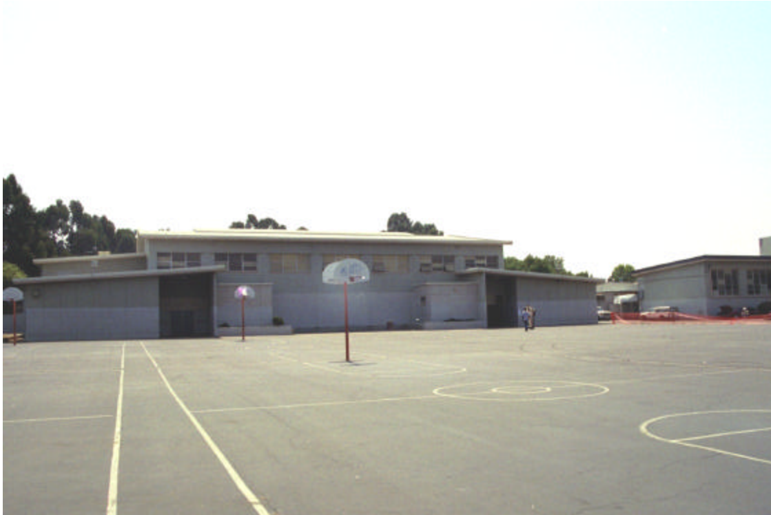
Figure 14: Gymnasium Building, exterior north wall
